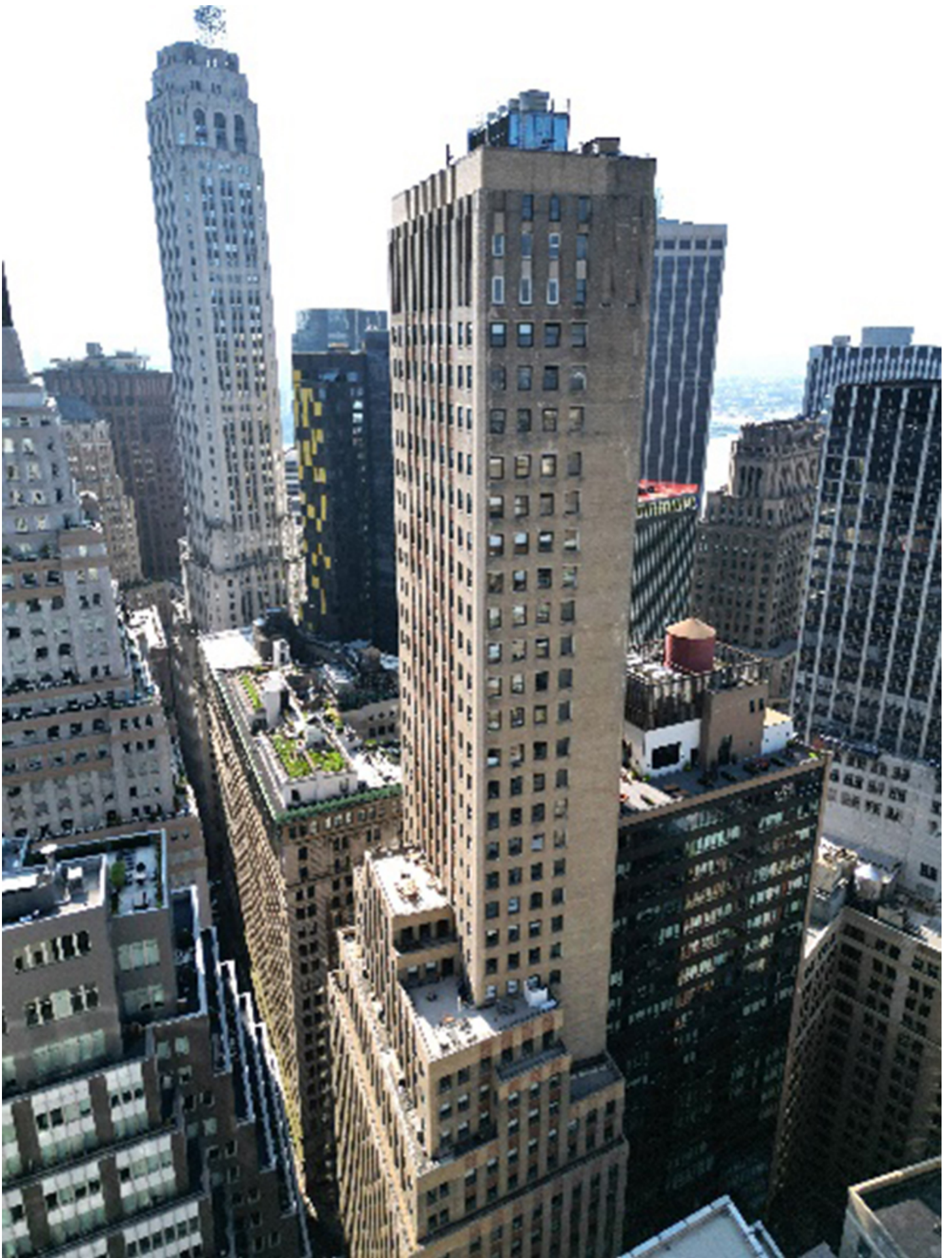
Manhattan, NY Central Construction is finishing an all-encompassing project at the historic Financial District office tower, 30 Broad St. For nearly two years, the work on the 50-story building has
