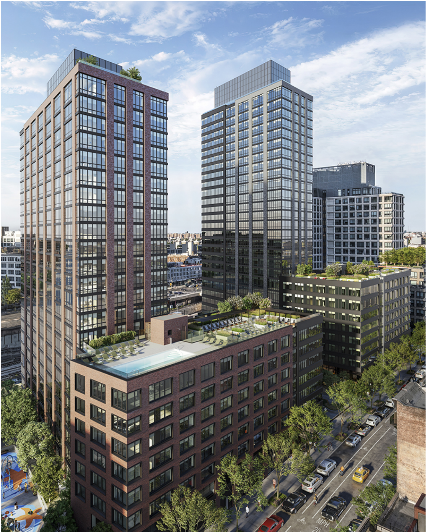
Brooklyn, NY According to developer TF Cornerstone (TFC) 595 Dean St. a mixed-use, two-tower development designed by Handel Architects has opened. Located in the Prospect Heights
