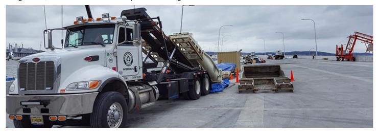
Concrete Washout System on-site for the Governor Mario M. Cuomo Bridge (Tappan Zee Bridge) that created a safer commuter route between Westchester and Rockland Counties and crosses the Hudson River at one of its widest points. During peak construction periods, over 35 patented Concrete Washout System's containers were utilized to prevent caustic concrete washout from entering the Hudson River.
