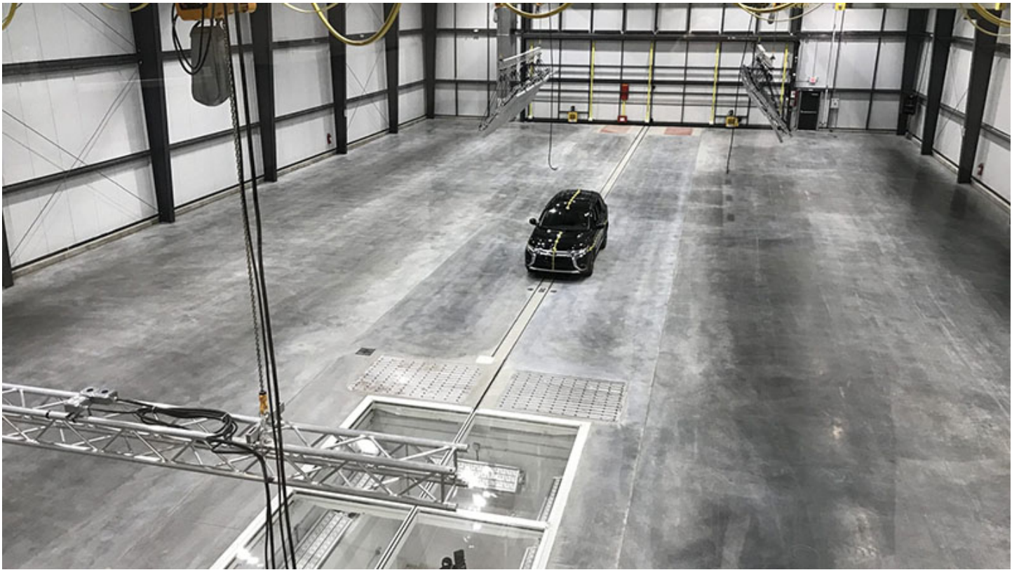
One of two indoor crash bays at the new Calspan facility, 4455 Genesee Street - Buffalo, NY
