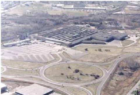
Salina Industrial Powerpark, 1 General Motors Drive - Salina, NY
