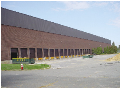
Forsgate property after renovation
