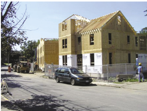
Row house #2 under construction.
