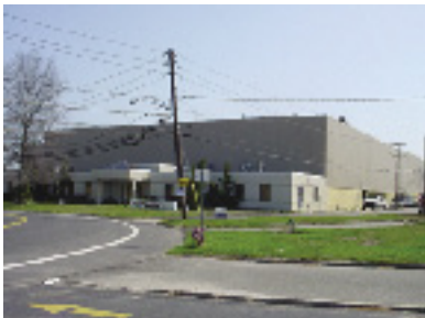
Sam Tell Co. site after Roof lifted to 35' clear
