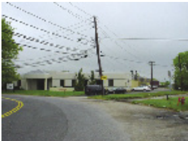
Sam Tell Co. site. Roof 14' clear
